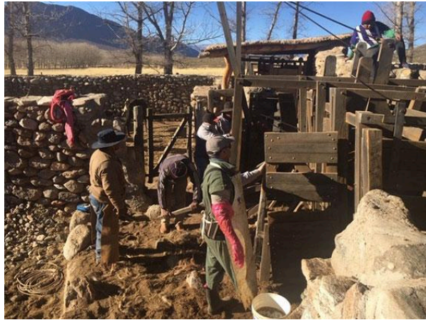
Working the chute
