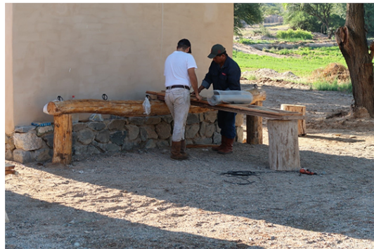
The carpenters at work
